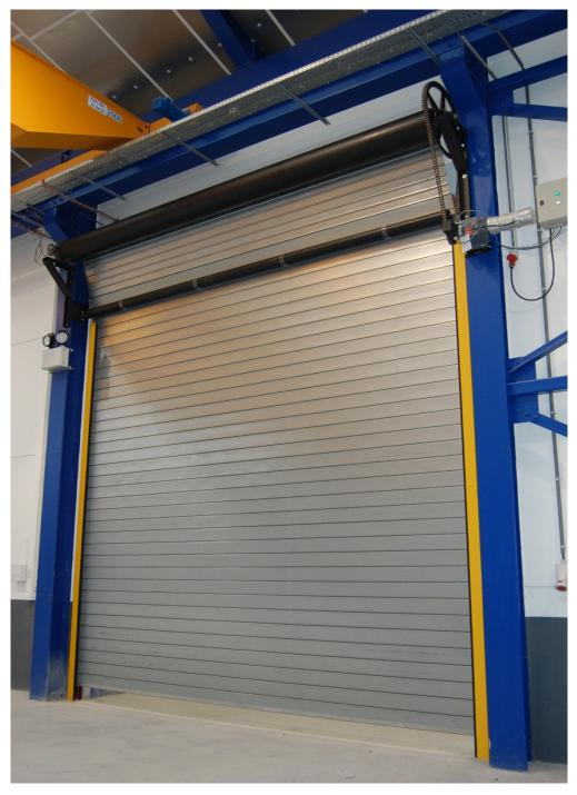
Automatic fire rolling doors are designed to separate the two fire sections and created the fire temporary barrier to prevent the spread of fire. Doors are not designed by their frequent use of weight as a normal door, their primary function is the closing in case of fire.
