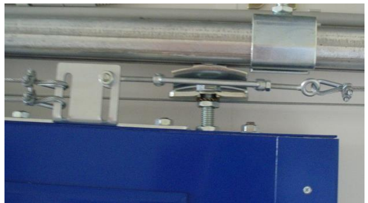
Door pull with screw turnbuckle
